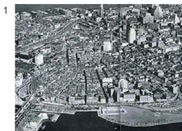
July 1958. Prior to Demolition
